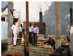
Construction at Raju Colony
