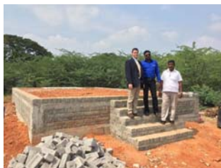
Construction at Madurai
