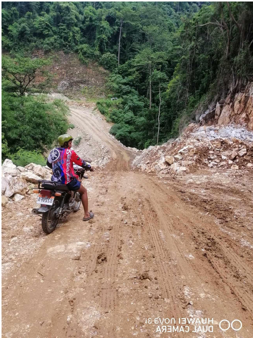
The slippery road going to Occidental Mindoro.
